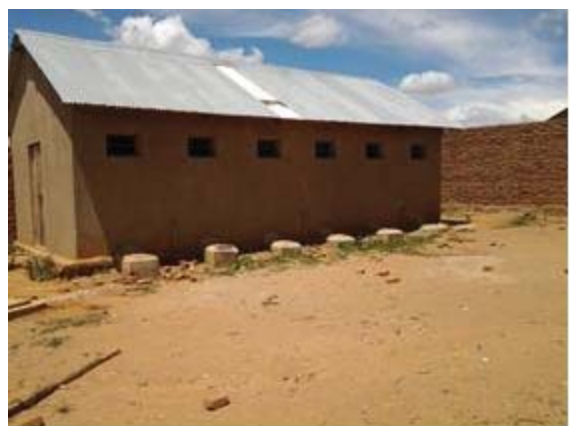
(b) Bathroom and Toilets
