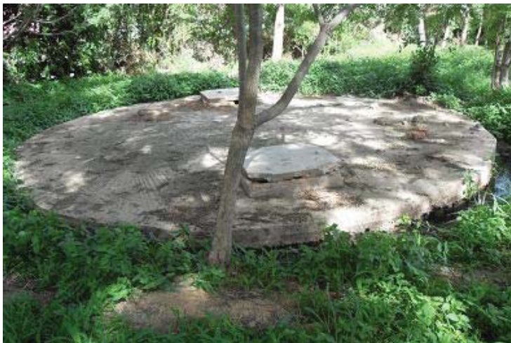
(a)The existing soak away pit
