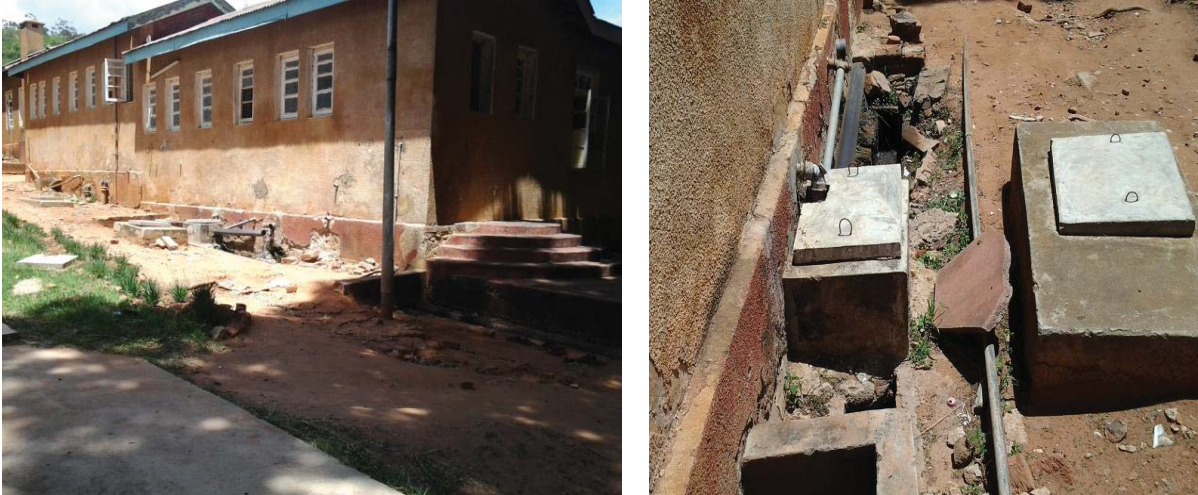
Figure 3.5: The old infrastructure of wastewater collection in toilets of LSS
