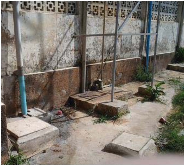
(a) Inspection chamber receiving water from washrooms of the dormitory at IGSS (b) Overflowing of chamber after bathing at IGSS
