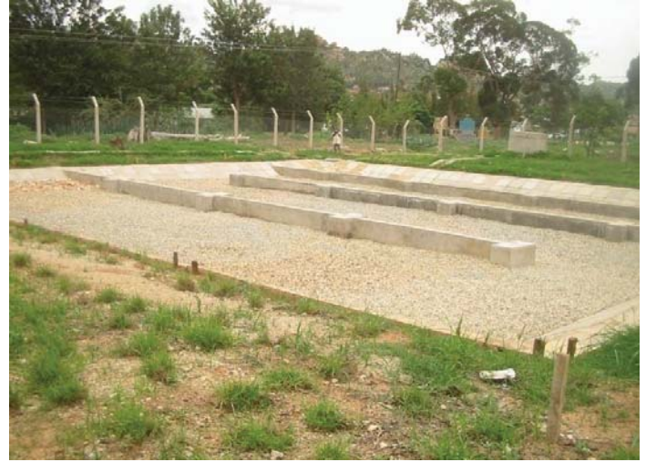
Figure 2. Conditions of Rehabilitated System at Kleruu
